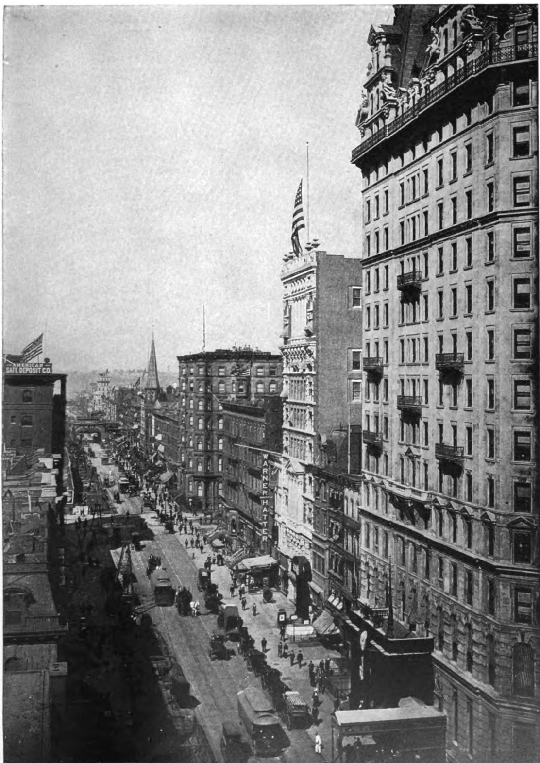
LOOKING WEST ON FORTY-SECOND STREET, NEW YORK. Hotel Manhattan on the right. One side of the street is torn up for subway construction.
